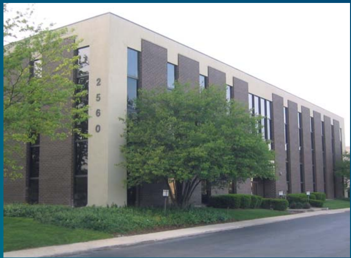
PULS facility located in St. Charles, Illinois
